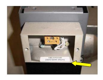
Position a Heater Electrical Warning "lightning" label, loose in the connection box.
